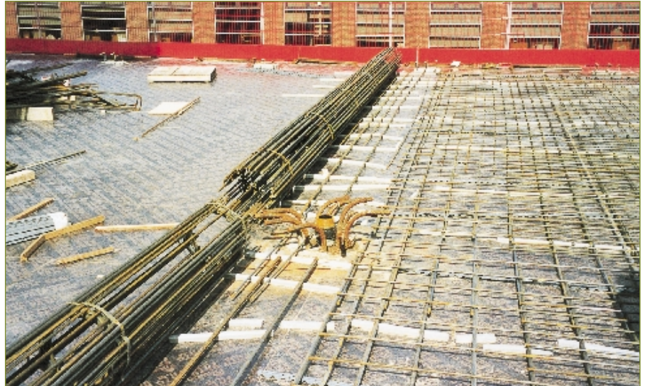
Figure 1: Reinforcing a flat slab using one-way spanning roll-out mats
