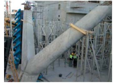
Completed raking V-column.
