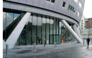
V-column complete at rear of building.
