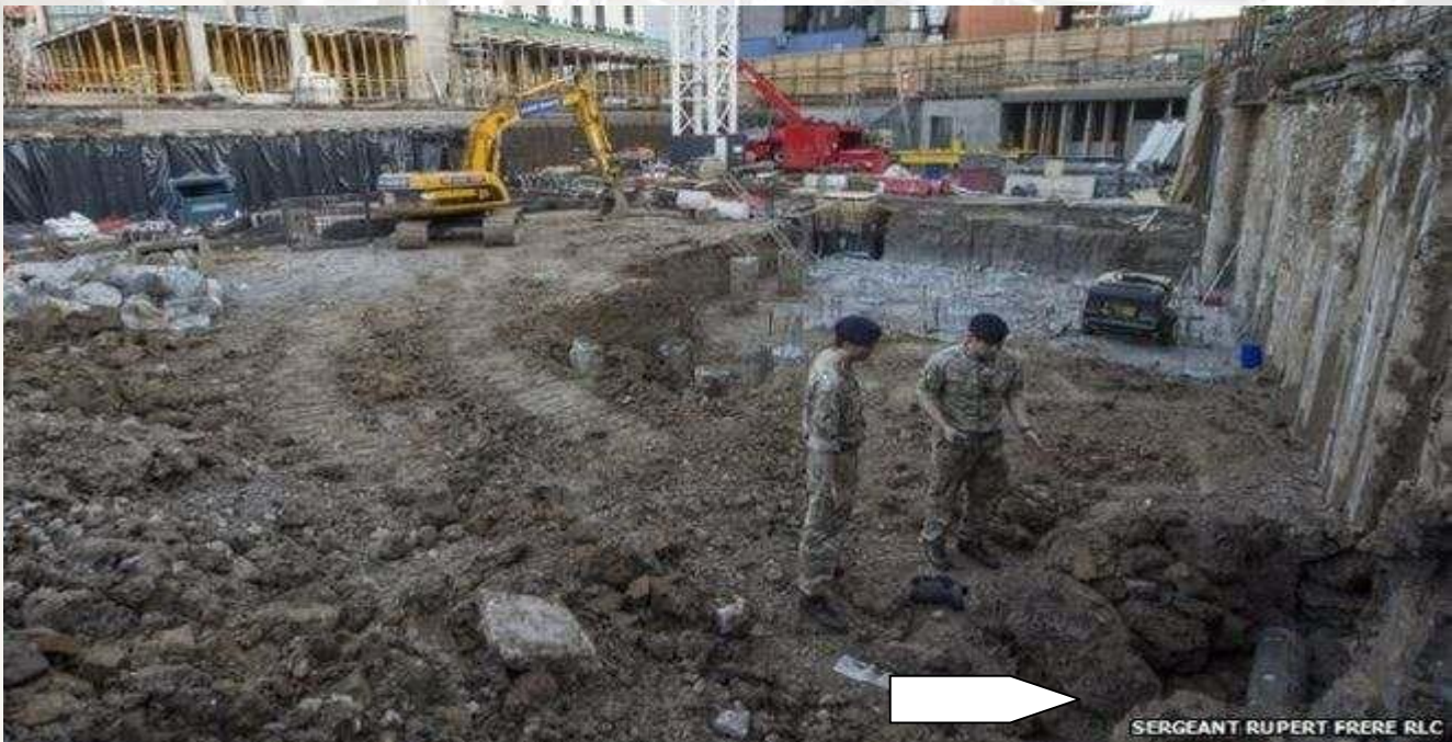
How close to Secant Piled Wall!!!
